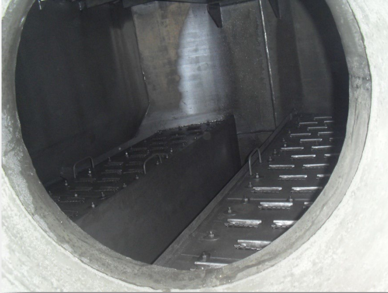
Interior view after cleaning
